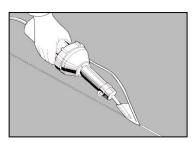
Weld with hot-air and Tarkett Speed Welding Nozzle. Carry out a test welding on a left-over piece before commencing work, to adjust speed and temperature.
